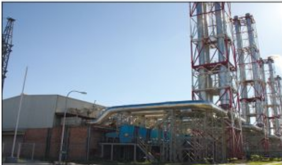
Our Bank Financed Project
